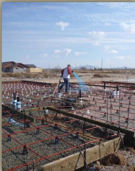
Termite pretreatment Image Credit: Ralph Morris, GRIC PCO
