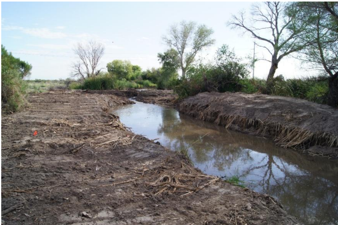
Figure 5 Pee Posh Wetlands Channel After Work
