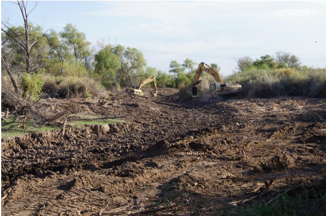
Figure 4 Sediment Removal in Pee Posh Wetlands
