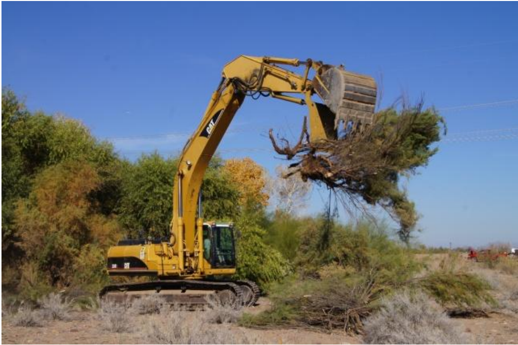
Figure 2 Saltcedar Removal - Root Ball Extraction
